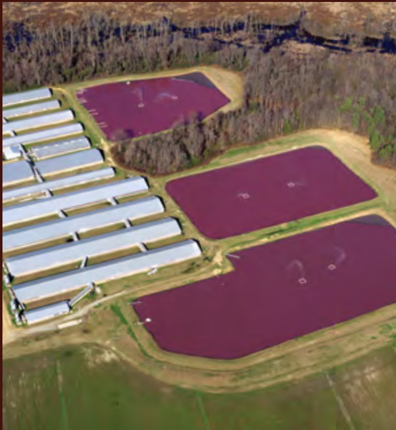
Massive facilities require massive waste management systems, like these treatment pools, which present a variety of environmental risks.
